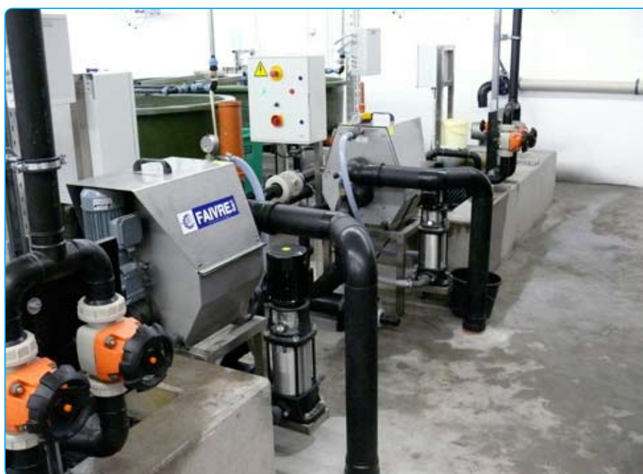
Drum filter model 1-40 with tank ( in sturgeon recirculation system )
